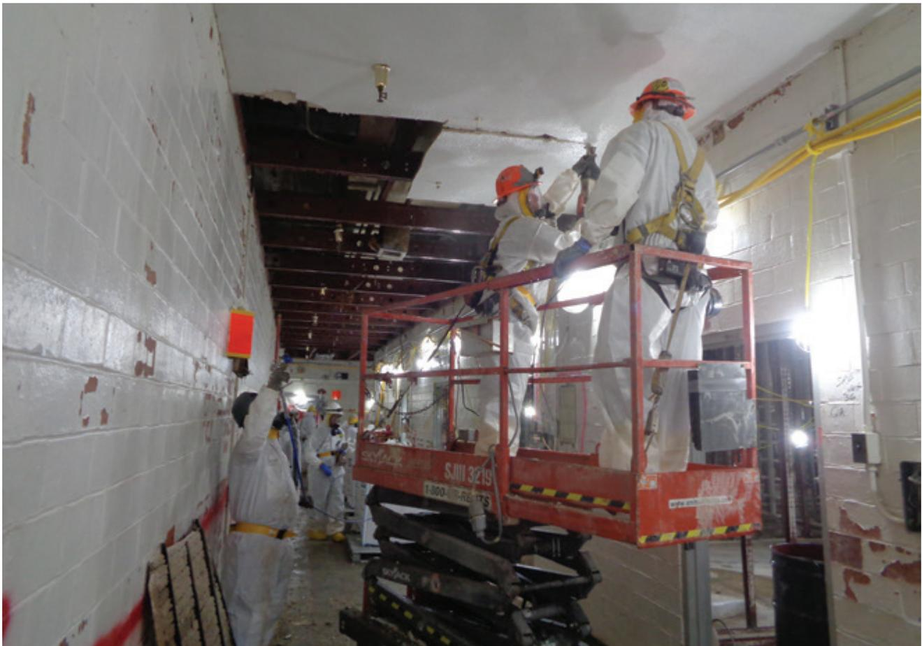
*Workers are removing asbestos in the Biology Complex*
