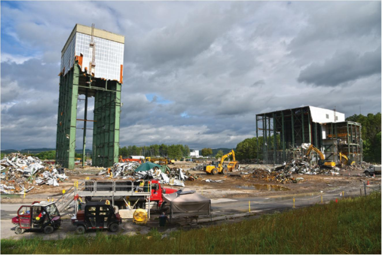
Demolition of the Centrifuge Complex removed the last super structure at ETPP. The demolition left behind a large slab (below), which workers began removing at the beginning of FY 2021.
