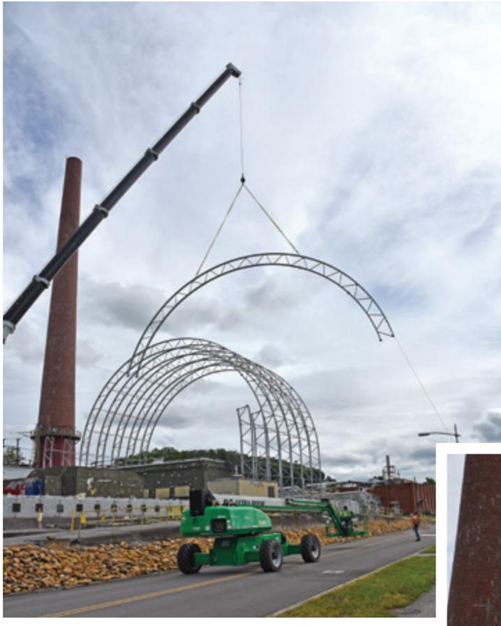
*UCOR constructed a protective tent over the 3026 facility to allow safe demolition of the hot cells*
