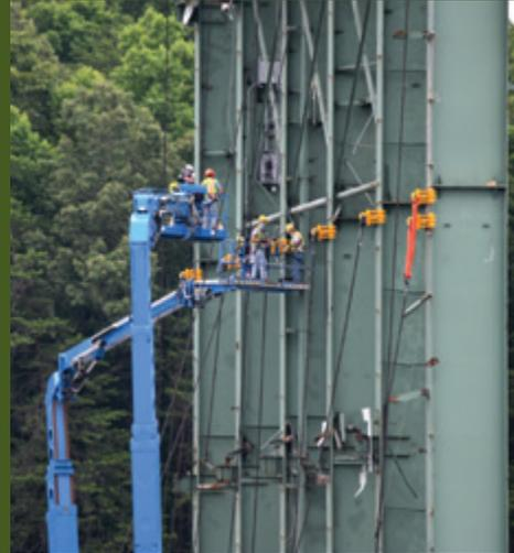
*The Centrifuge Complex tower pulldown was accomplished by large winches (below). Workers above attach the lines to the tower.*
