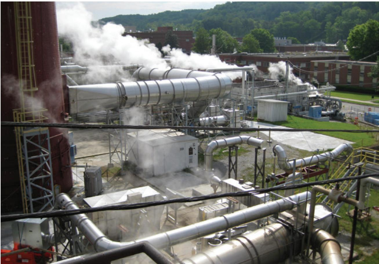
Treatment System at Building 3608. The new system installation was completed, and it is now removing cesium and strontium from LGWO wastewater. As a result, the Rad Process Waste Treatment Complex (Building 3544) that has exceeded its design life is in
