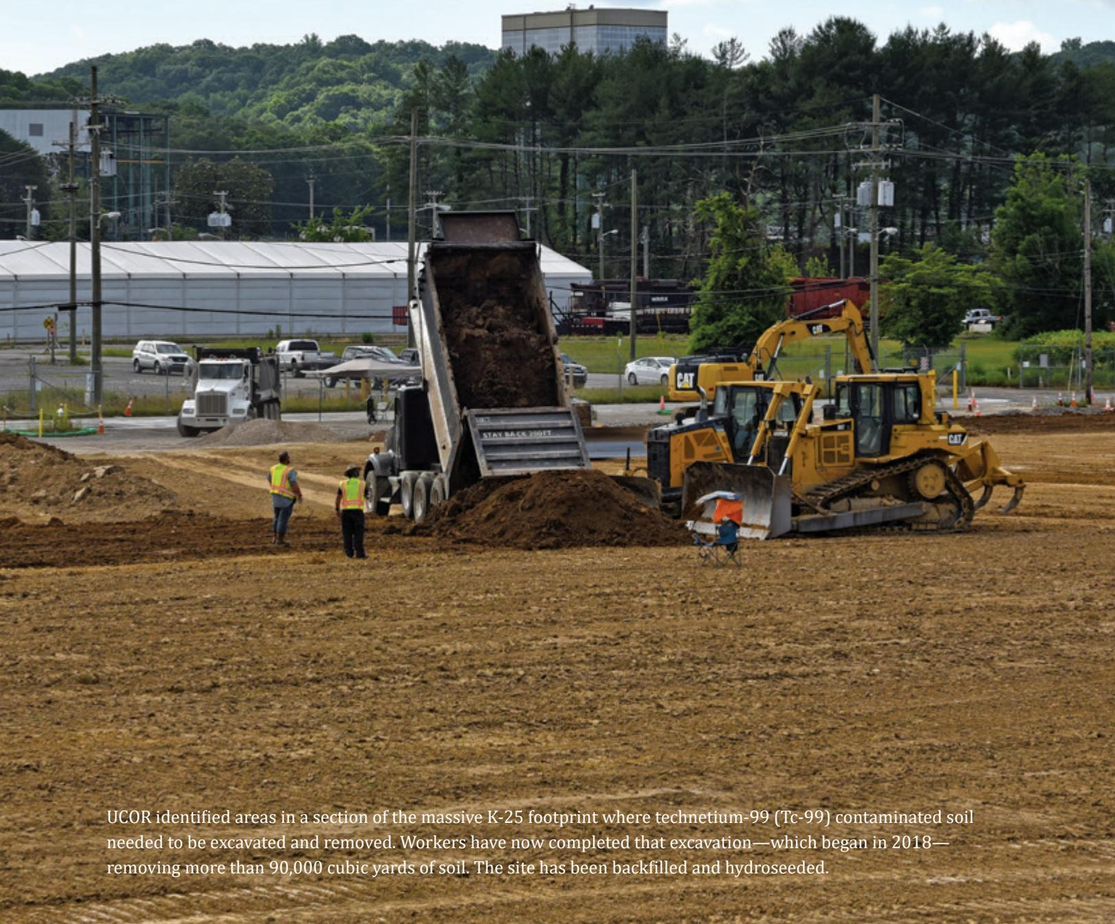
UCOR identified areas in a section of the massive K-25 footprint where technetium-99 (Tc-99) contaminated soil needed to be excavated and removed. Workers have now completed that excavation—which began in 2018—removing more than 90,000 cubic yards of soil. The site has been backfilled and hydroseeded.
