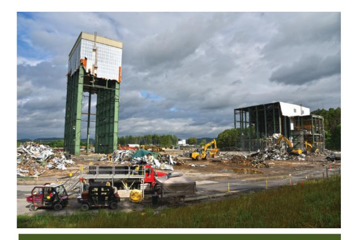
Demolition of the Centrifuge Complex removed the last super structure at ETTP. The demolition left behind a large slab (below), which workers began removing at the beginning of FY 2021.
